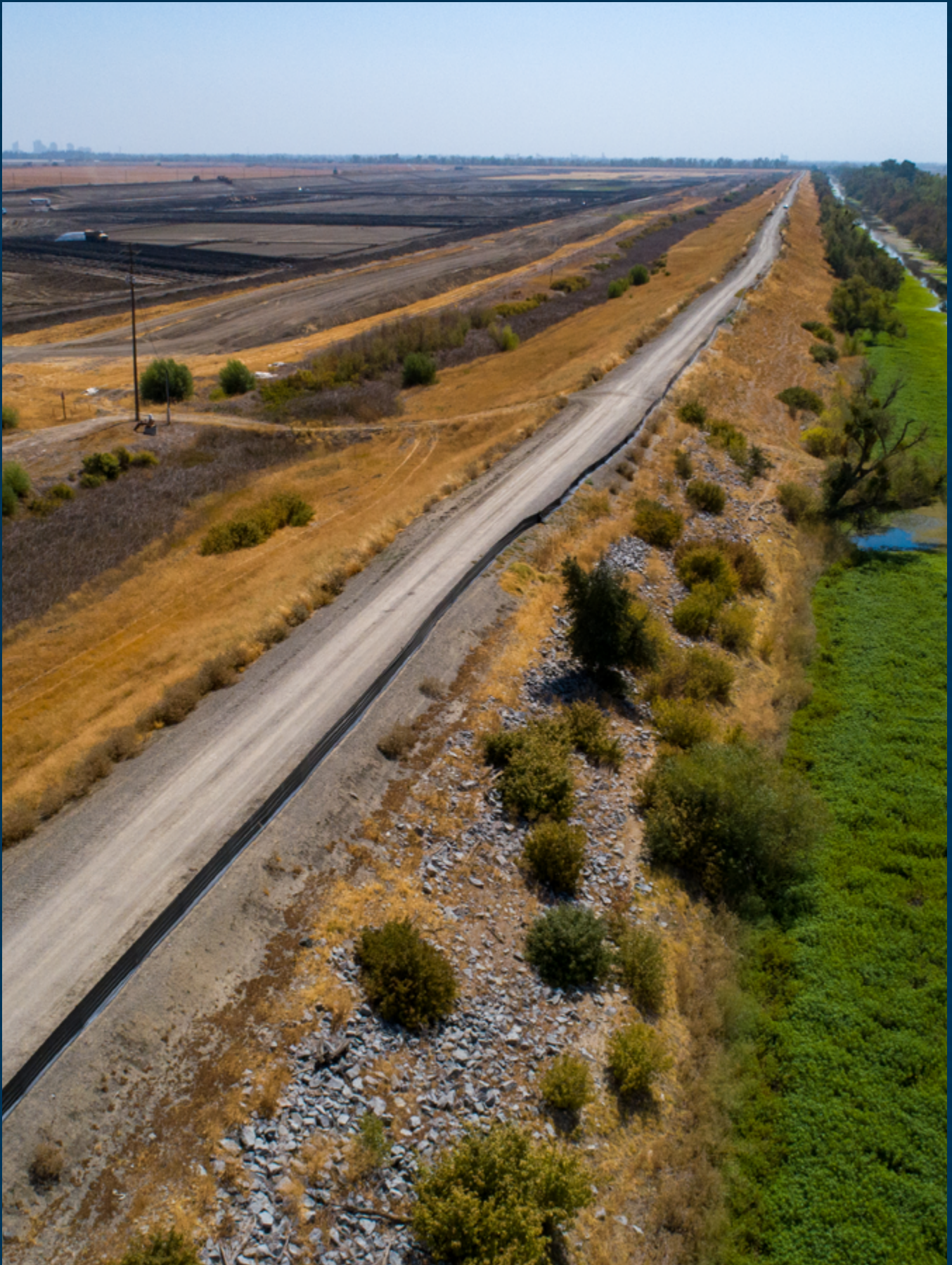
The California Department of Water Resources is constructing setback levees along the Sacramento and Yolo bypasses as part of the Lower Elkhorn Basin Levee Setback project. Photo taken August 31, 2021.
