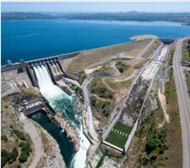
Completed Folsom Lake Dam Modification Project in 2019. Photo provided by California Department of Water Resources.
