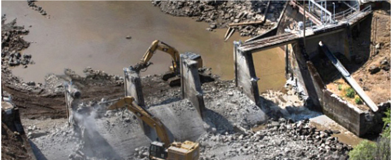
Copco Dam 2 removal was completed in July 2023.
