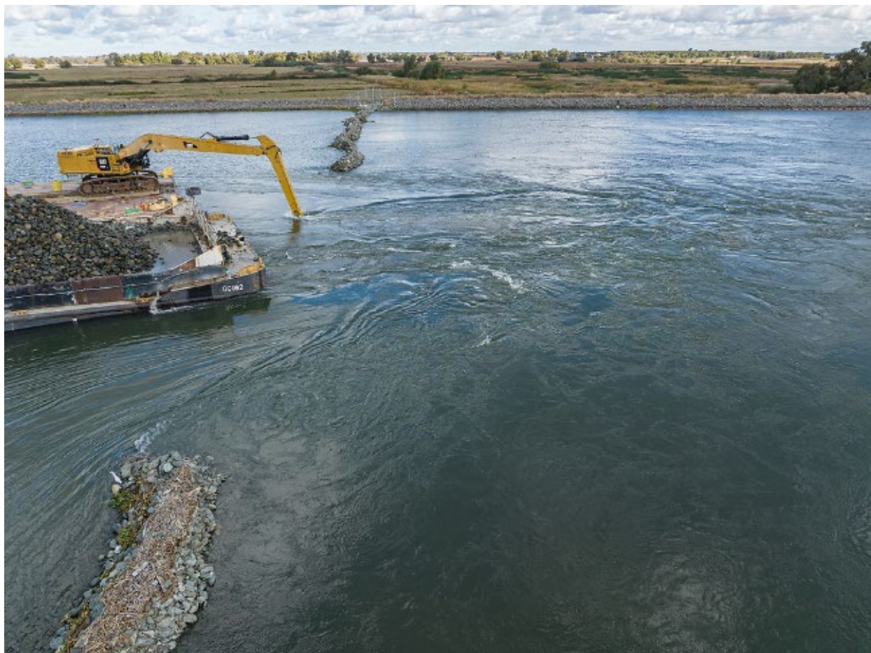
Figure 1.3-1 Removal of the temporary emergency drought barrier in West False River.
