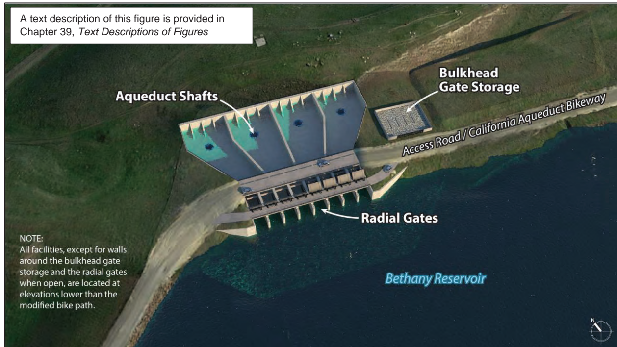
5 6 Figure 3-34. Bethany Reservoir Discharge Structure
