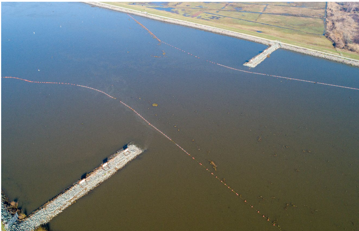
Figure 2. The 2021 Barrier with notch removed to allow fish passage
